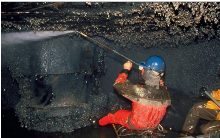
Figure G.22 Masked workers use a water jet to clear zebra mussels clogging the walls of the pump room of Detroit Edison's power station in Michigan, USA. Not only do zebra mussels encrust water pipes and pump rooms, but they also excrete a corrosive substance.
